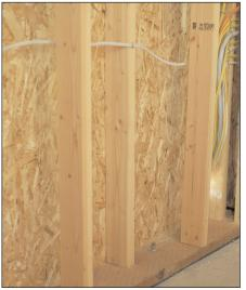
Above, the Rose House, owned by Eldon Haines and Linda Rose, when finished will be an accessory dwelling unit which generates more electricity than it will use. The Rose House uses a structural insulated panel system at the roof, a staggered stud system, at left, at the walls and special foundation insulation minimizing details. temperature changes.
